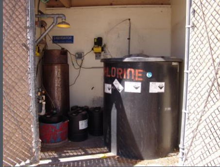
Replace CO2 Tank Replace Acid Tank
