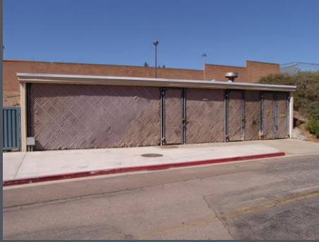
Existing Pool Equipment Room
