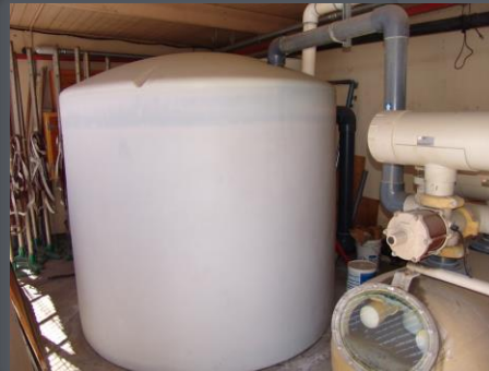
Replace pool water holding tank Replace old piping
