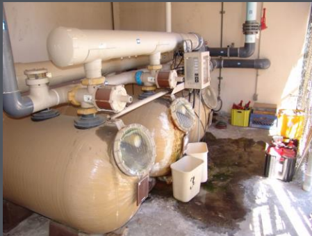
Replace existing leaking sand filter tank backwash system
